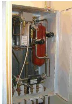
*Vital Energy – Hydraulic Interface Unit (indirect Mini-plate heat exchanger)*
