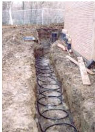
*Fig. 6.6 - Typical geothermal horizontal sub-soil pipes*
