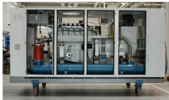
*Fig 7.2 Internal working of CHP unit*
